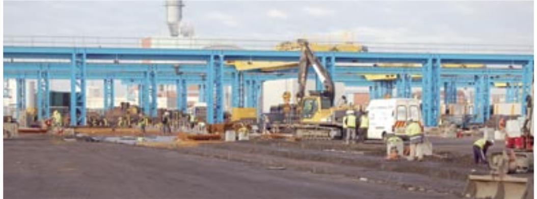
The underground foundations are now complete after having set a unique set of construction challenges for the builders, Mitchell Design & Construction. Hundreds of concrete piles 16 metres long had to be driven into the ground through the sturdy remains of the old Brighton 'B' Power Station coal yard. The obstructions encountered included a complete underground
